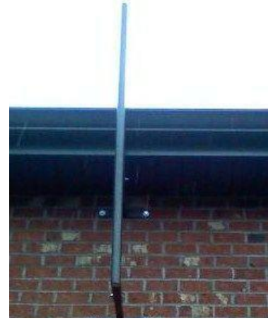
Cranky Post Type 2 – Gutter Mount
