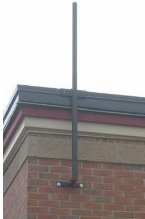
Cranky Post Type 3 Adjustable Bottom Legs
